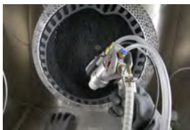
Blast gun being used in hand-held manual operation
